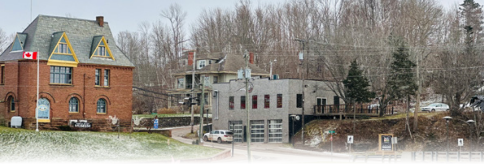
The Town of Three Rivers' municipal water and sewer services are concentrated in Montague and municipal sewer services in Georgetown. Photo: Montague, Three Rivers
