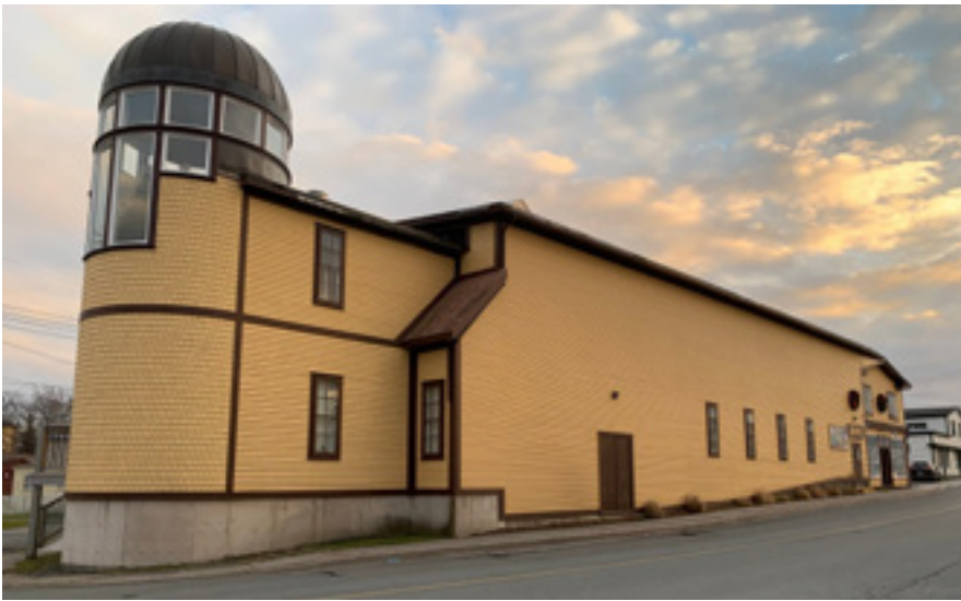
After an extensive renovation, the Garrick Theatre reopened in 2010 as a social enterprise, with operations subsidized by the Town of Bonavista. Photo: Garrick Theatre
