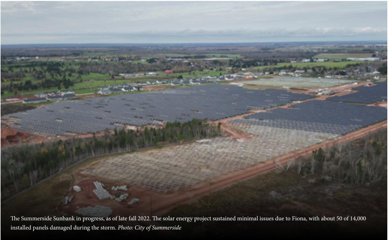
The Summerside Sunbank in progress, as of late fall 2022. The solar energy project sustained minimal issues due to Fiona, with about 50 of 14,000 installed panels damaged during the storm. *Photo: City of Summerside*
